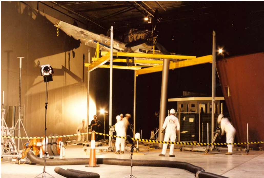
Figure 6. Aircraft at correct height for display, waiting for support column to be rolled into position. The aircraft was then lowered onto the column for final fixing.
