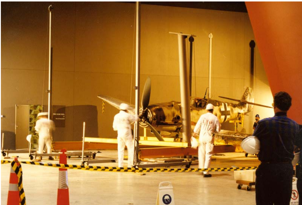
Figure 4. Site cleared of miscellaneous items ready for lift. Note mast hoists at each major beam end – these are the lifting mechanisms for the aircraft. The crane does not give a sufficient level of control and precision to ensure the safety of the object, staff and exhibition infrastructure so is not used for this purpose.
