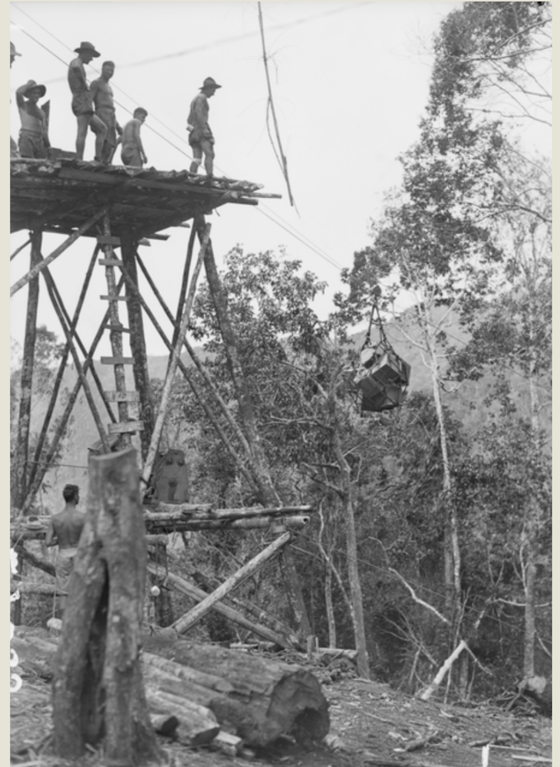
Flying fox constructed by 2/6th Field Company, Royal Australian Engineers, to carry supplies to the start of the track to Uberi, Papua. Photograph by Thomas Fisher, October 1942. AWM 027033
