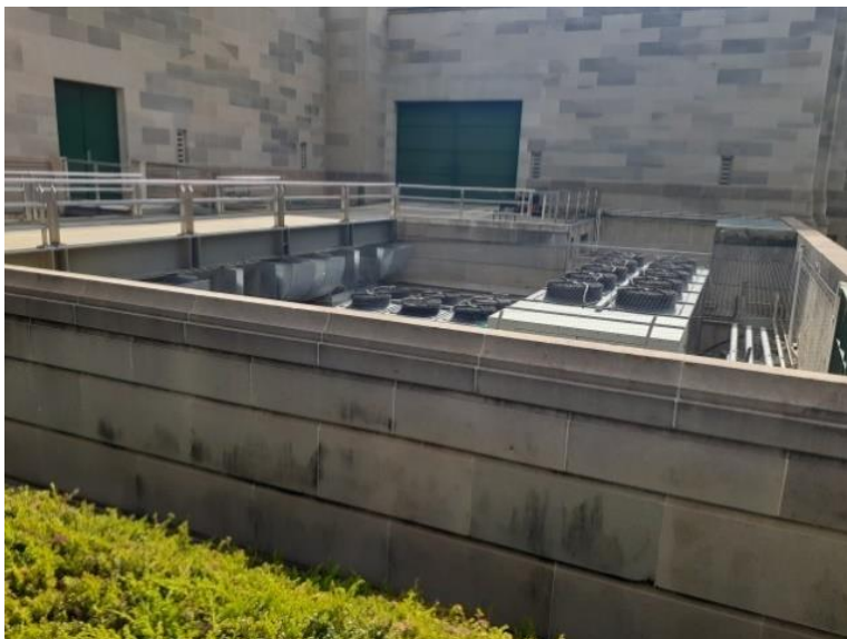
Figure 7.4 – Unenclosed air cooler enclosure to rear of the Main Building
