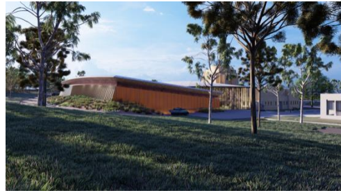
View of Anzac Hall from north-west
