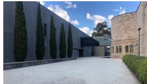
View of current Main Building rear from the west
