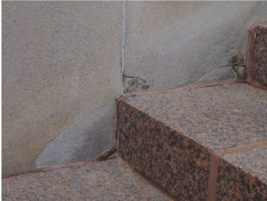
Figure 18 Localised exfoliation to ashlar at the abutment of the granite steps. Replacement or repair of the sandstone will be required on reconstruction of the bastion wing walls. (Photo: Jasper Swann, 12 February 2020)
