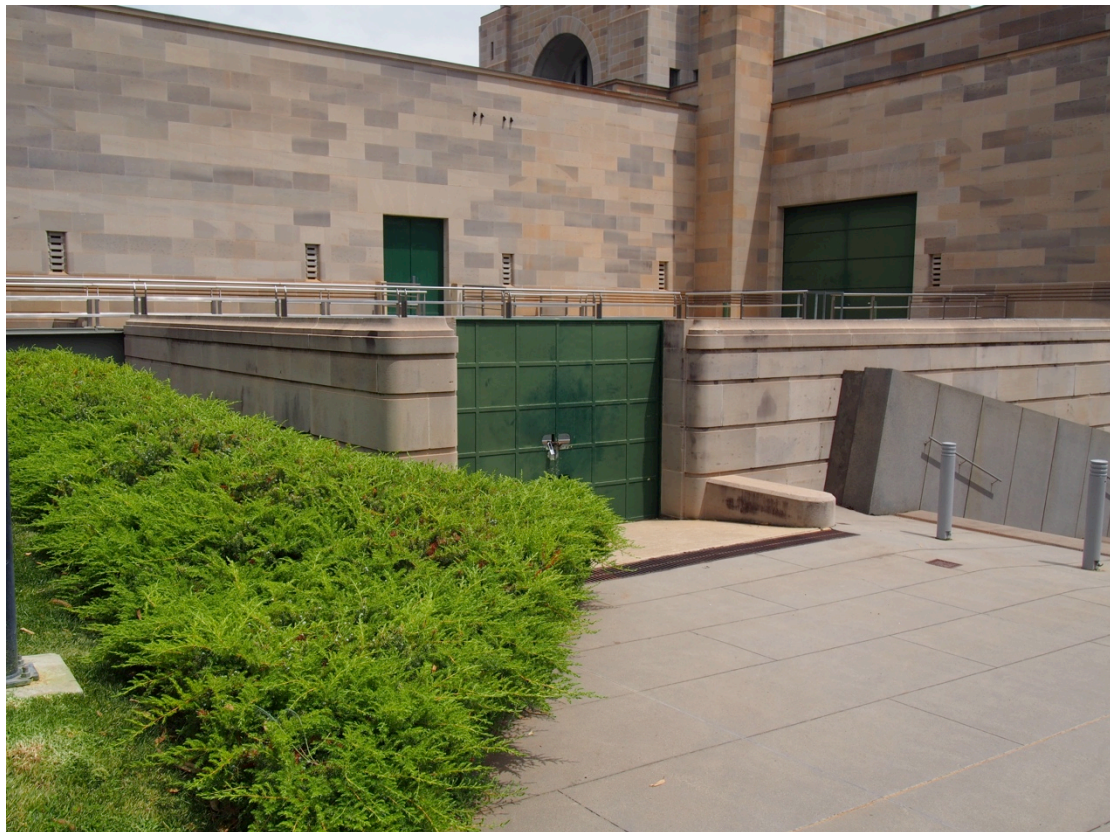
Figure 20 The lower walls around the plant room are to be partially demolished. Careful dismantling and salvage of the sandstone in these walls is recommended, as there is potential for reuse in the reconstruction of the bastion wing walls at the front entrance. (Photo: Jasper Swann, 12 February 2020)
