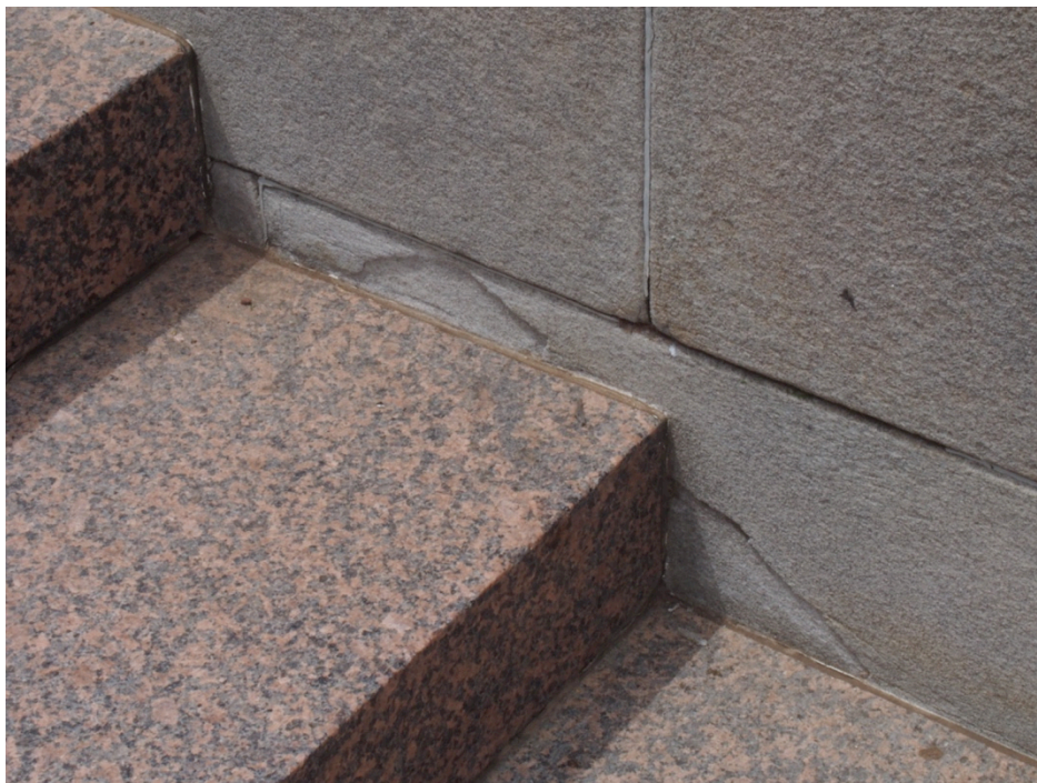
Figure 16 Cracking at edge of copings on the western bastion wall. This type of deterioration will not withstand dismantling and will require repair, either with mortar repair or hairline indent on reconstruction. (Photo: Jasper Swann, 12 February 2020)
