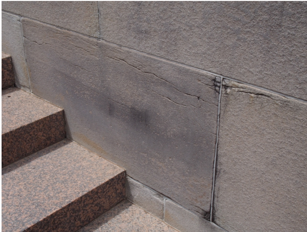
Figure 10 Stone in west elevation of eastern wing wall in poor condition. This stone will require replacement on reconstruction. (Photo: Jasper Swann, 12 February 2020)
