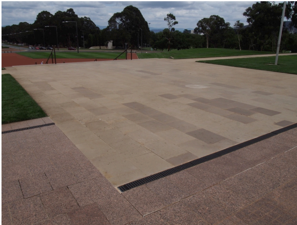
Figure 21 Sandstone paving to forecourt. (Photo: Jasper Swann, 12 February 2020)
