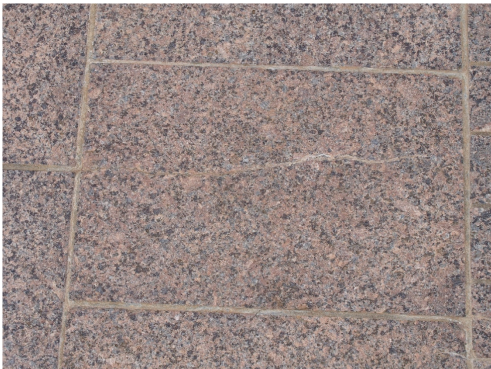
Figure 4 One of several cracked granite pavers to forecourt. (Photo: Jasper Swann, 12 February 2020)
