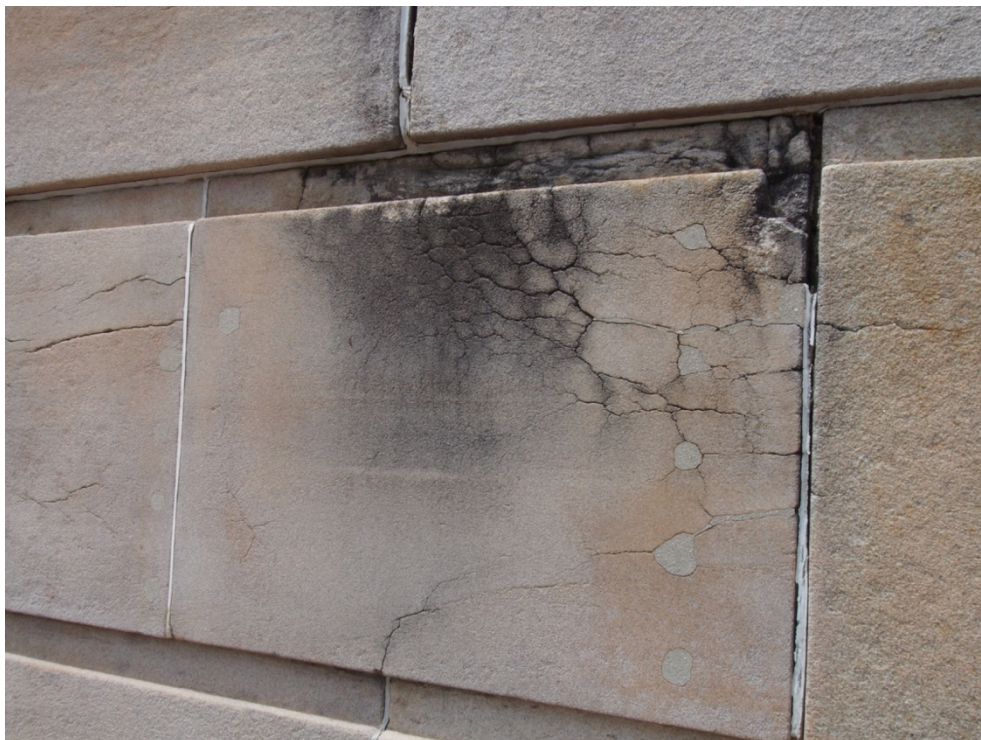
Figure 10 Stone in west elevation of eastern wing wall in poor condition. This stone will require replacement on reconstruction. (Photo: Jasper Swann, 12 February 2020)
