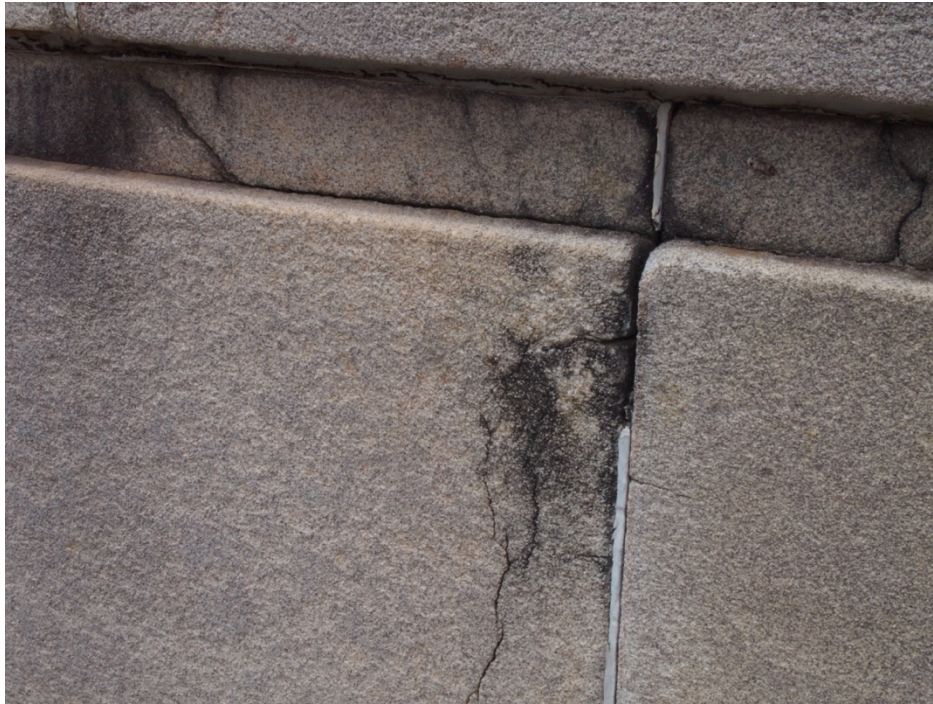
Figure 14 Cracking at edge of ashlar on the eastern bastion wall. This type of deterioration will not withstand dismantling and will require repair, either with mortar repair or hairline indent on reconstruction. (Photo: Jasper Swann, 12 February 2020)
