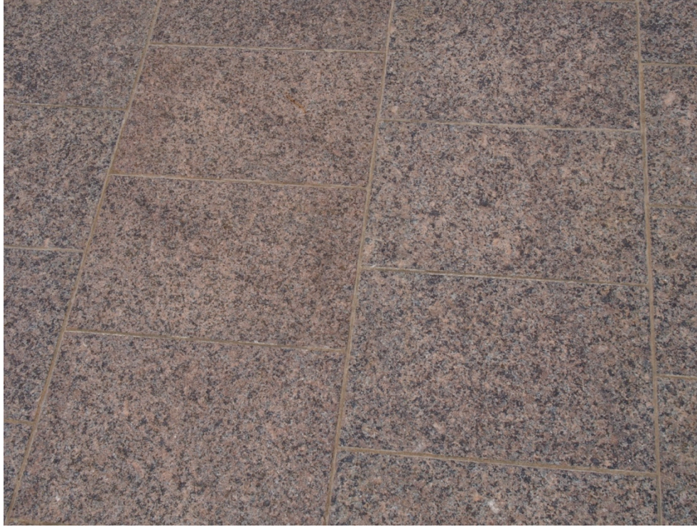
Figure 2 450mm x 300mm granite pavers to forecourt. (Photo: Jasper Swann, 12 February 2020)
