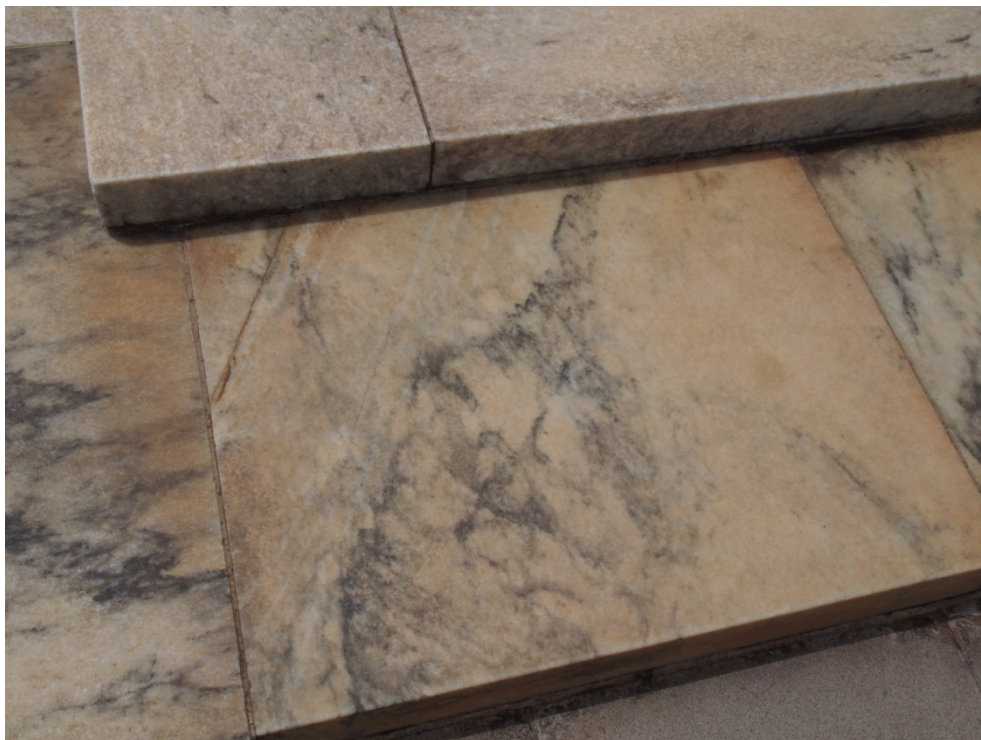
Figure 28 Cracking in marble step (top left corner), likely to break when dismantling. (Photo: Jasper Swann, 12 February 2020)
