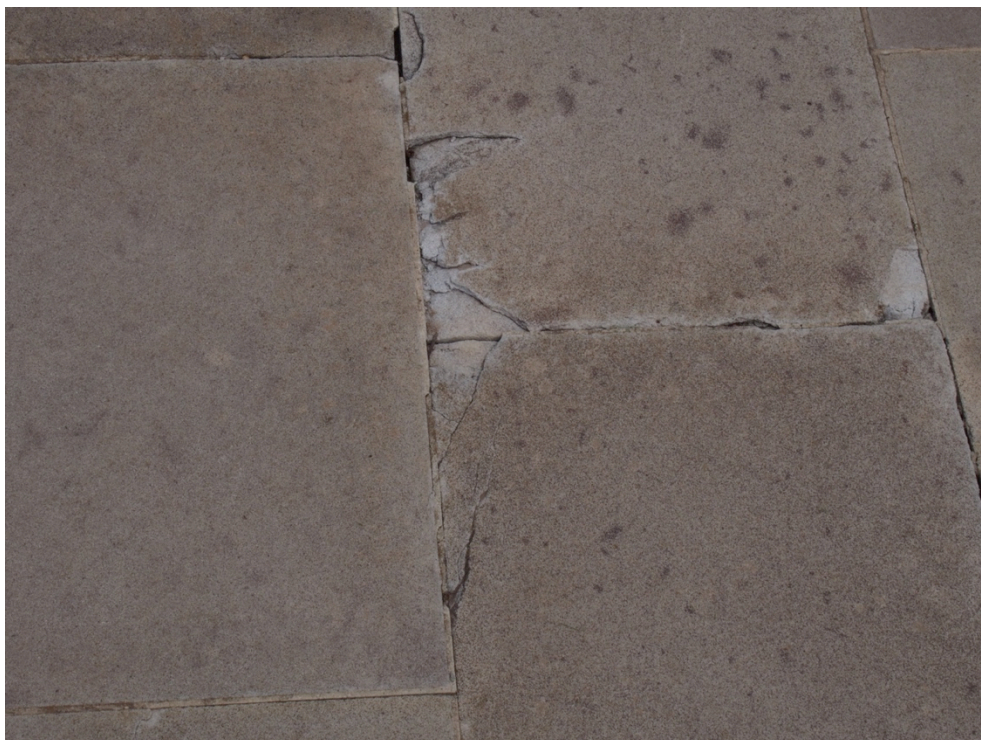
Figure 24 Localised damage to sandstone paving. The majority, however, is in good condition. (Photo: Jasper Swann, 12 February 2020)
