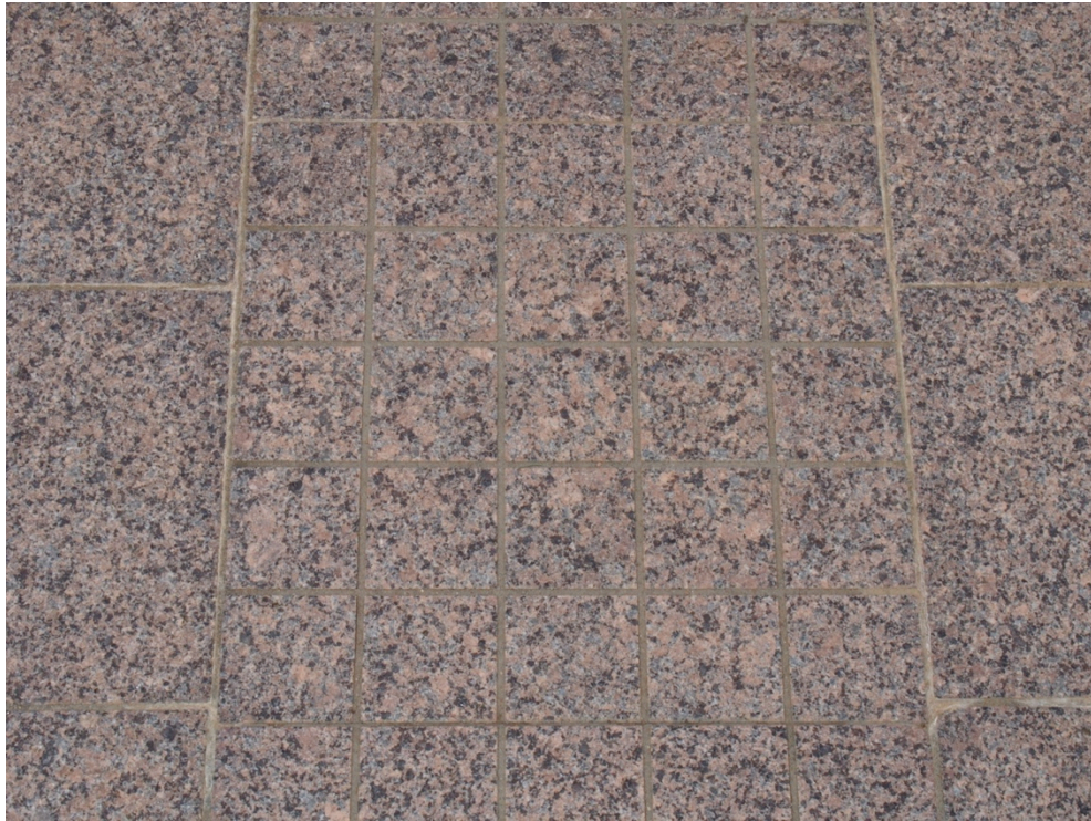
Figure 3 450mm x 450mm grid-scored granite paver to forecourt. (Photo: Jasper Swann, 12 February 2020)
