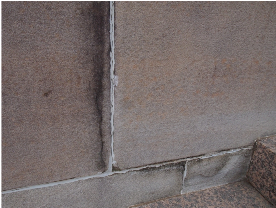
Figure 14 Cracking at edge of ashlar on the eastern bastion wall. This type of deterioration will not withstand dismantling and will require repair, either with mortar repair or hairline indent on reconstruction. (Photo: Jasper Swann, 12 February 2020)
