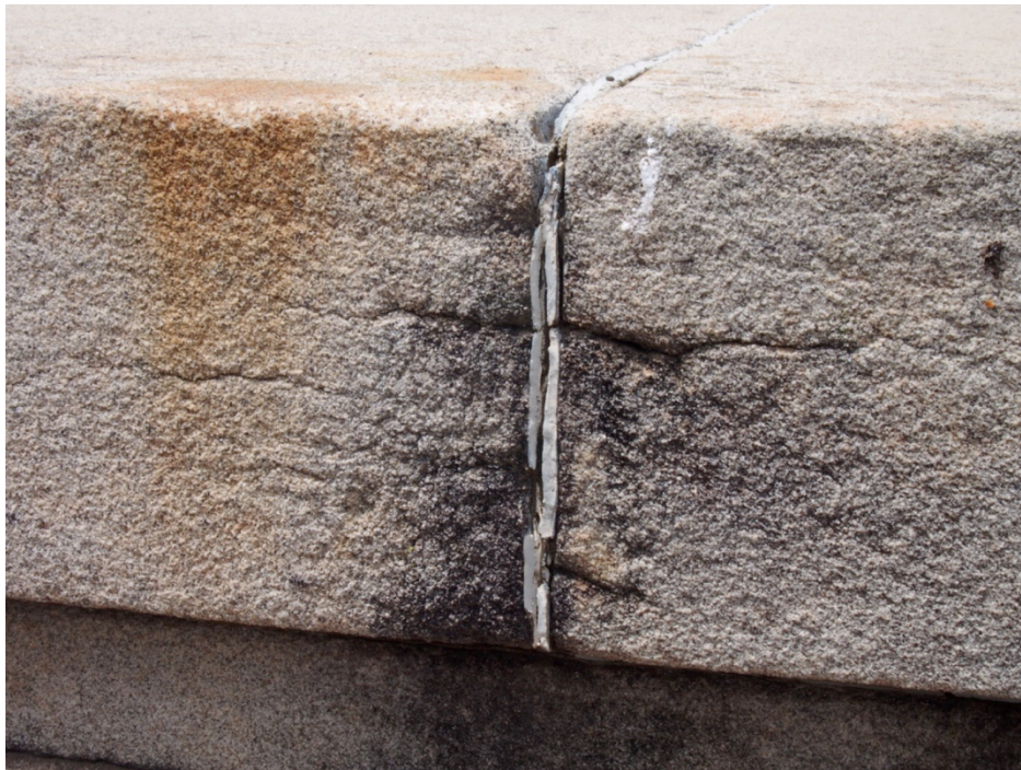
Figure 16 Cracking at edge of copings on the western bastion wall. This type of deterioration will not withstand dismantling and will require repair, either with mortar repair or hairline indent on reconstruction. (Photo: Jasper Swann, 12 February 2020)
