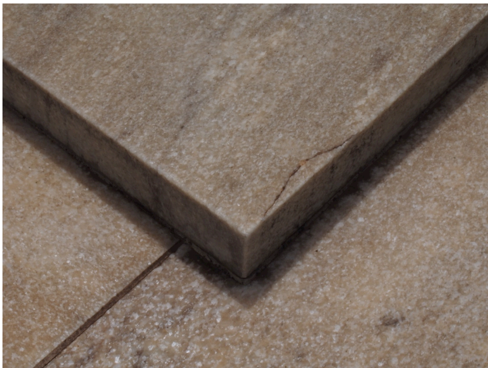
Figure 30 Cracking to leading edge of marble step requiring glue repair prior to dismantling. (Photo: Jasper Swann, 12 February 2020)
