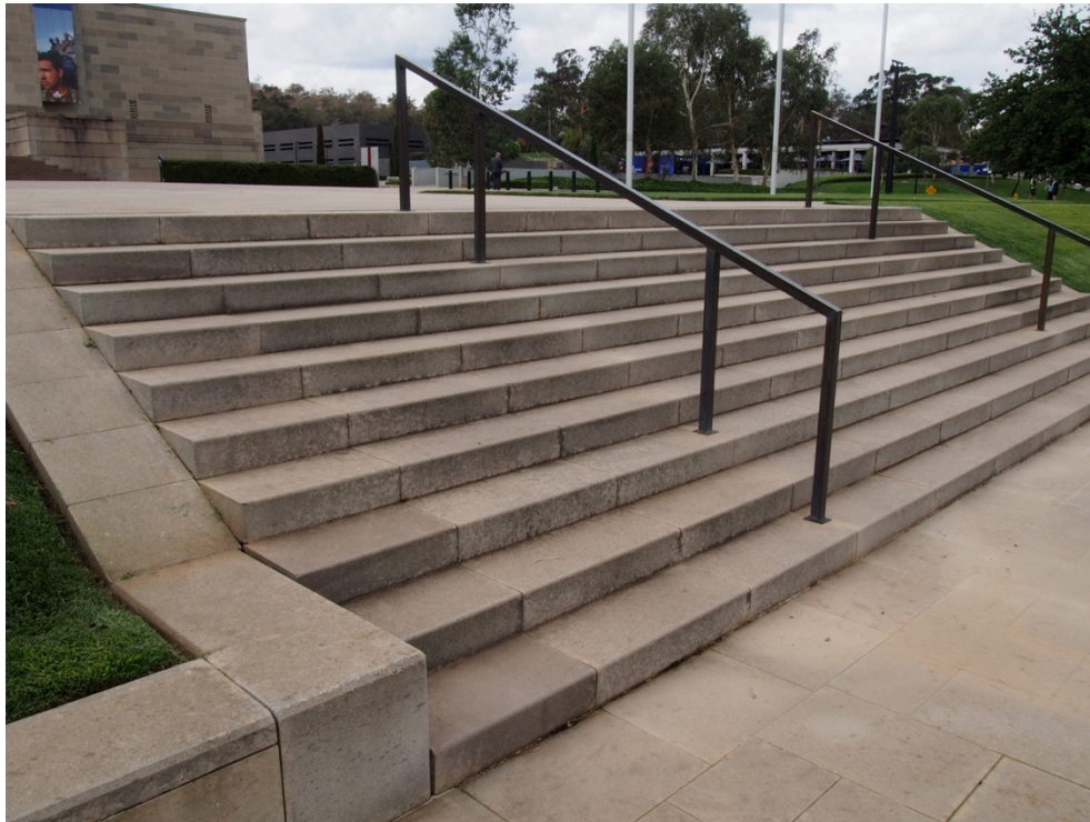
Figure 25 Wondabyne sandstone step treads to lower forecourt. Steps are in good condition. (Photo: Jasper Swann, 12 February 2020)
