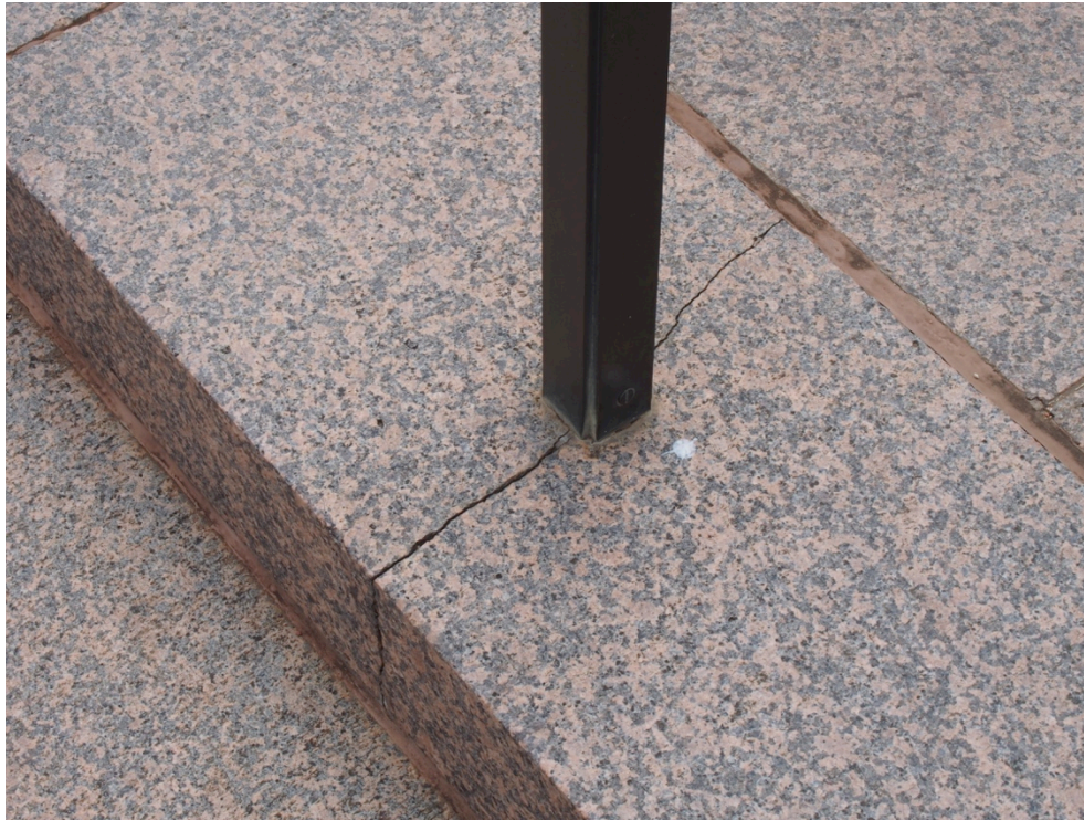
Figure 5 Cracked granite step tread to forecourt steps. (Photo: Jasper Swann, 12 February 2020)
