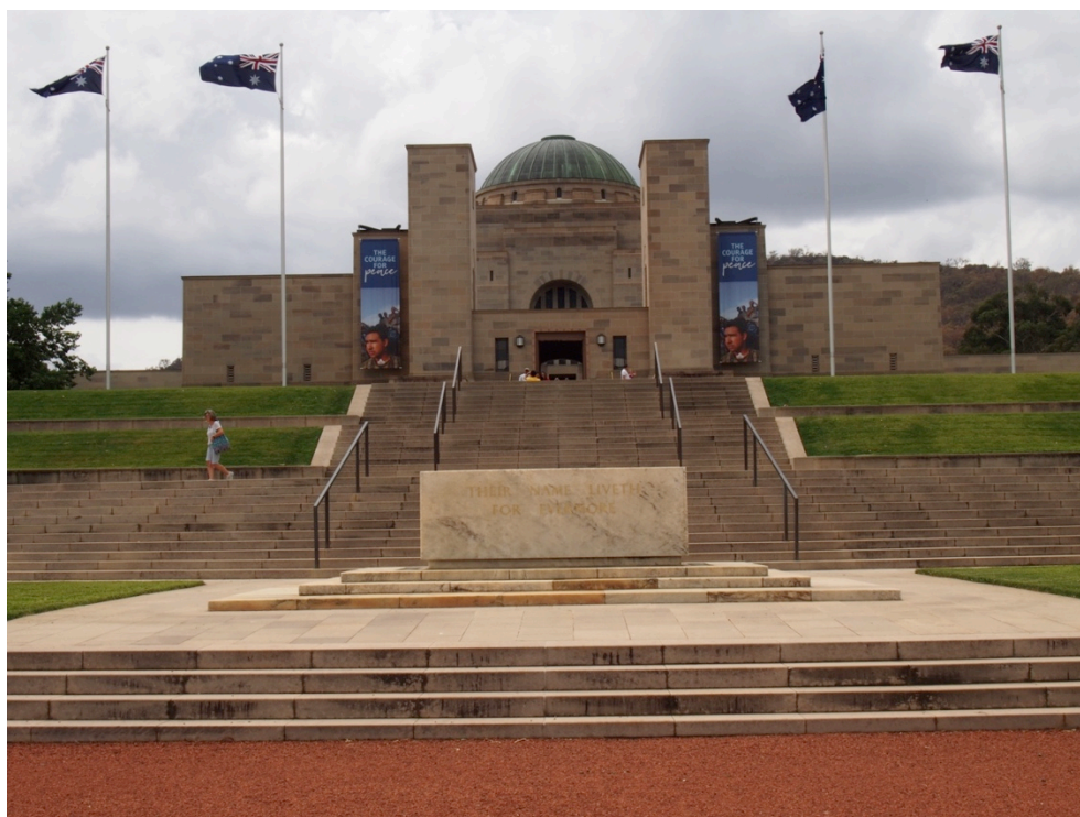
Figure 26 Three tiers of Wondabyne sandstone steps (seen behind the Stone of Remembrance), all in good condition. (Photo: Jasper Swann, 12 February 2020)
