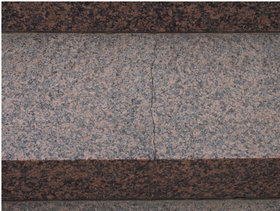
Figure 6 Cracked granite step tread to forecourt steps. (Photo: Jasper Swann, 12 February 2020)
