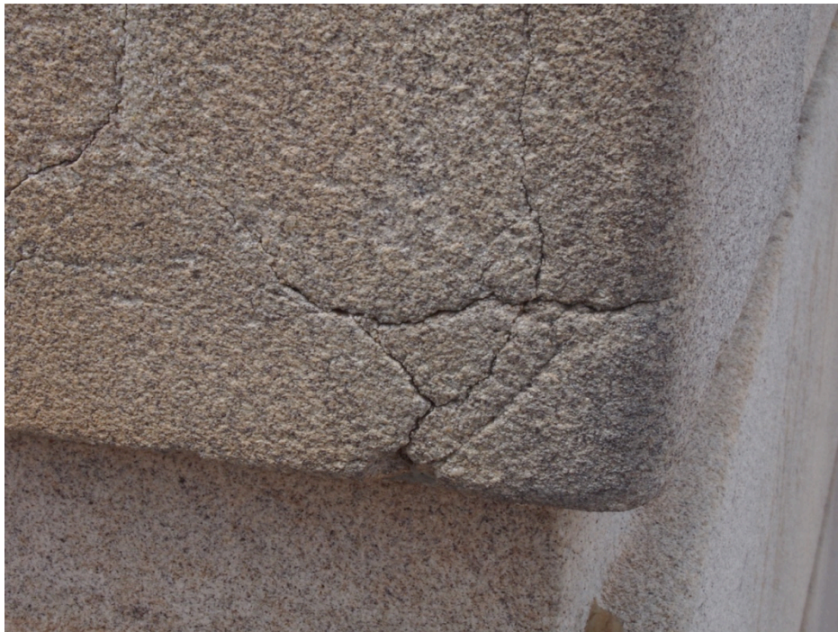
Figure 12 Stone in west elevation of western wing wall in poor condition. This stone will require replacement on reconstruction. (Photo: Jasper Swann, 12 February 2020)
