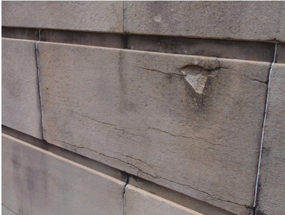
Figure 12 Stone in west elevation of western wing wall in poor condition. This stone will require replacement on reconstruction. (Photo: Jasper Swann, 12 February 2020)
