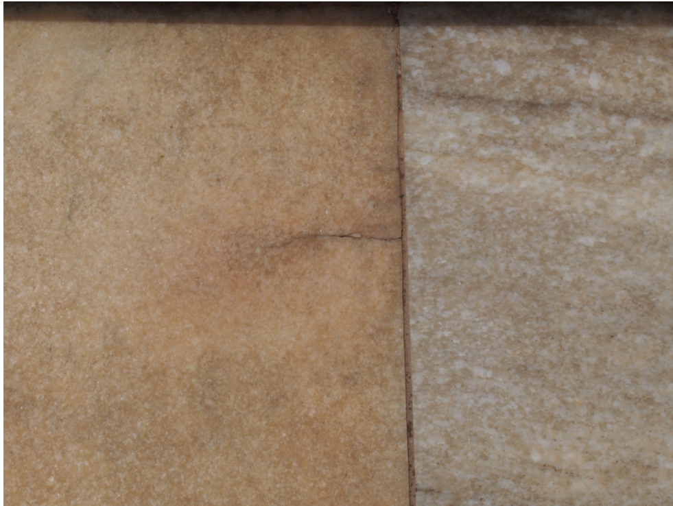
Figure 29 Cracking either side of joint in marble step course. (Photo: Jasper Swann, 12 February 2020)
