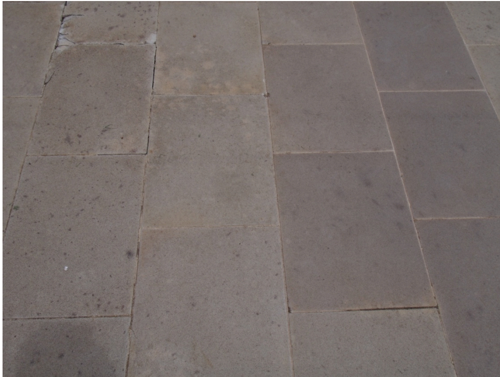
Figure 23 600mm x 420mm Wondabyne sandstone paving to the forecourt. (Photo: Jasper Swann, 12 February 2020)
