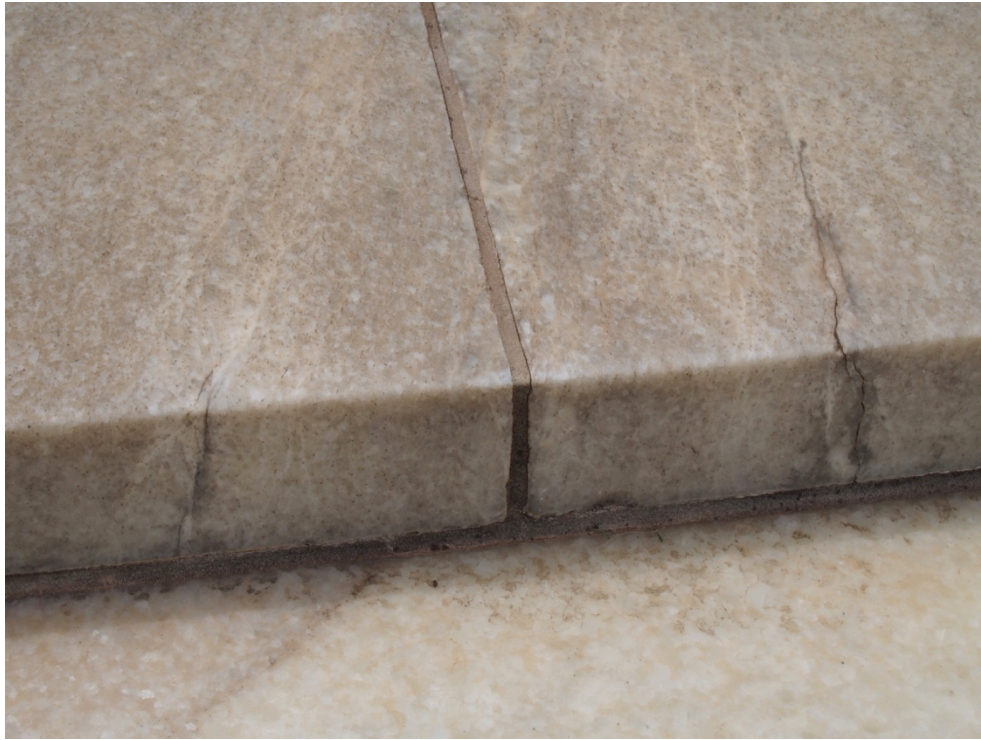
Figure 31 Cracking in marble step likely to break during dismantling. (Photo: Jasper Swann, 12 February 2020)
