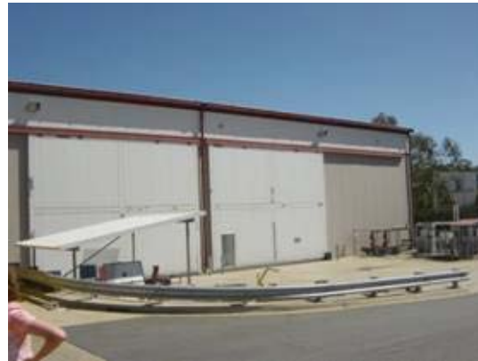
Figure 11 Treloar C from the rear, at the junction with Treloar B, built 1992.
