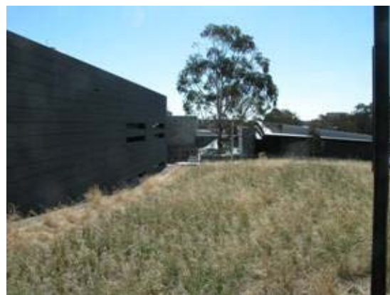
Figure 7 The northern elevation of the CEW Bean building softened by a grassed embankment.
