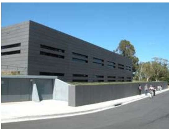
Figure 6 CEW Bean Building located to the east of the main complex.
