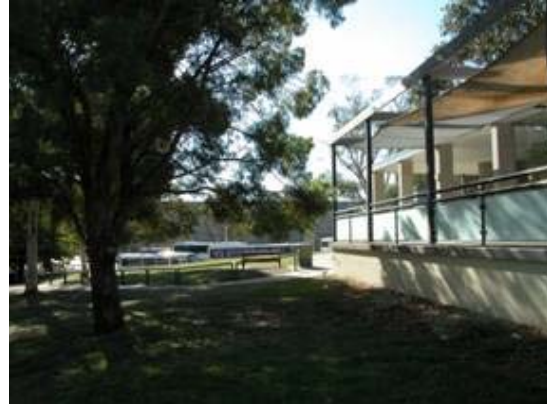
Figure 9 Recent verandah structure at the front of the Outpost Café.
