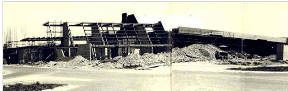
Construction of Annex A, 23 October 1978
