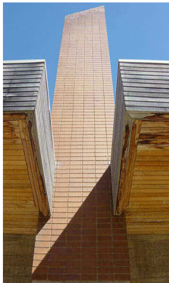
Vertical elements of the building provide balance to the overlapping horizontal planes.
