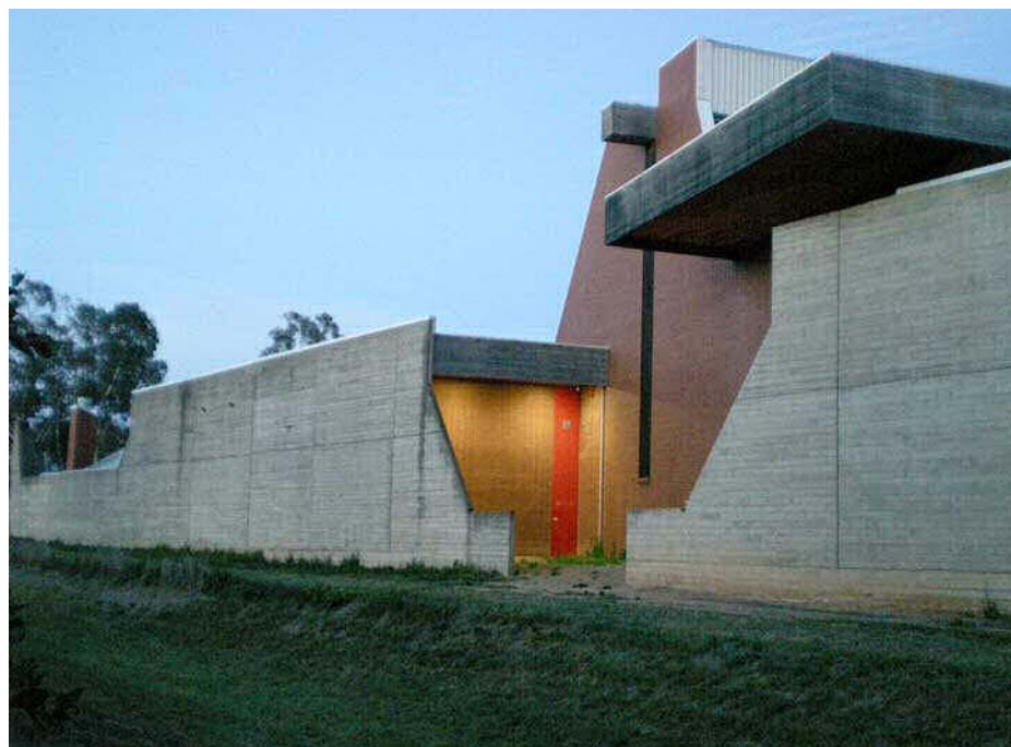
Northern elevation of Annex A, October, 2007.
