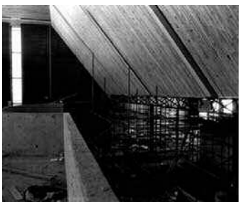
Clerestory windows provide natural light.
