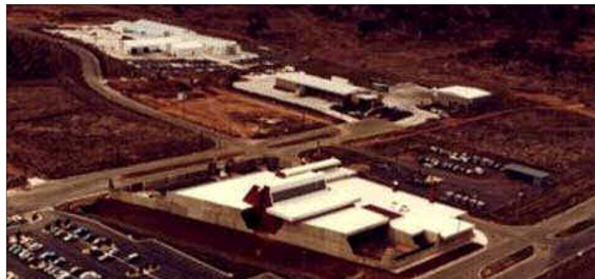
Aerial photograph of Annex A, looking NE, September 1979
