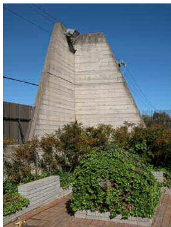
Component of the high off-form concrete security wall.
