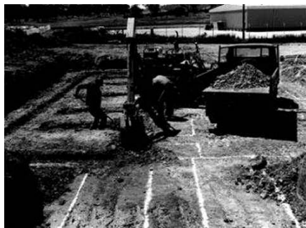
Preparing the site of the refrigerated vaults, November 1978. 21
