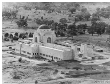
The landscape under construction. 3
