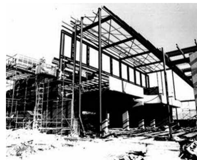
Annex A under construction. 22
