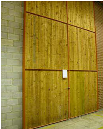
Custom designed sliding bay doors.
